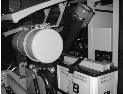
A. Hydraulic tank
